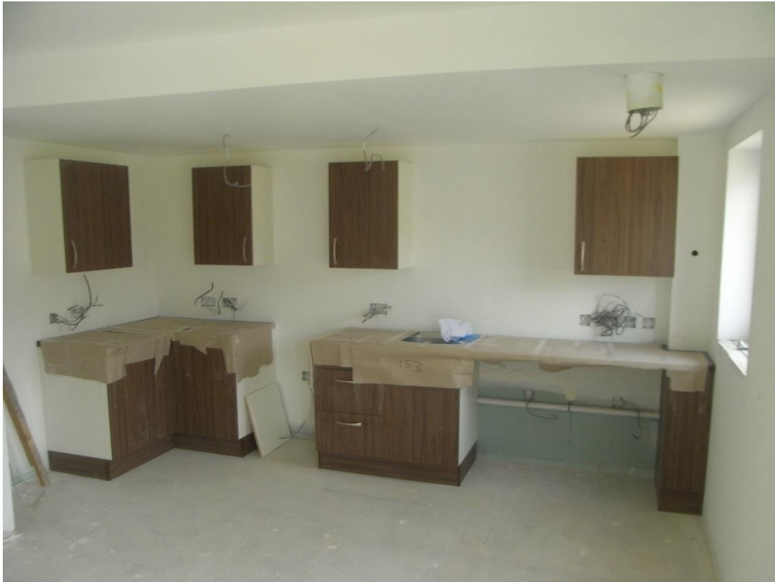
Block 5 – Kitchen fittings installation (28.09.2021)
