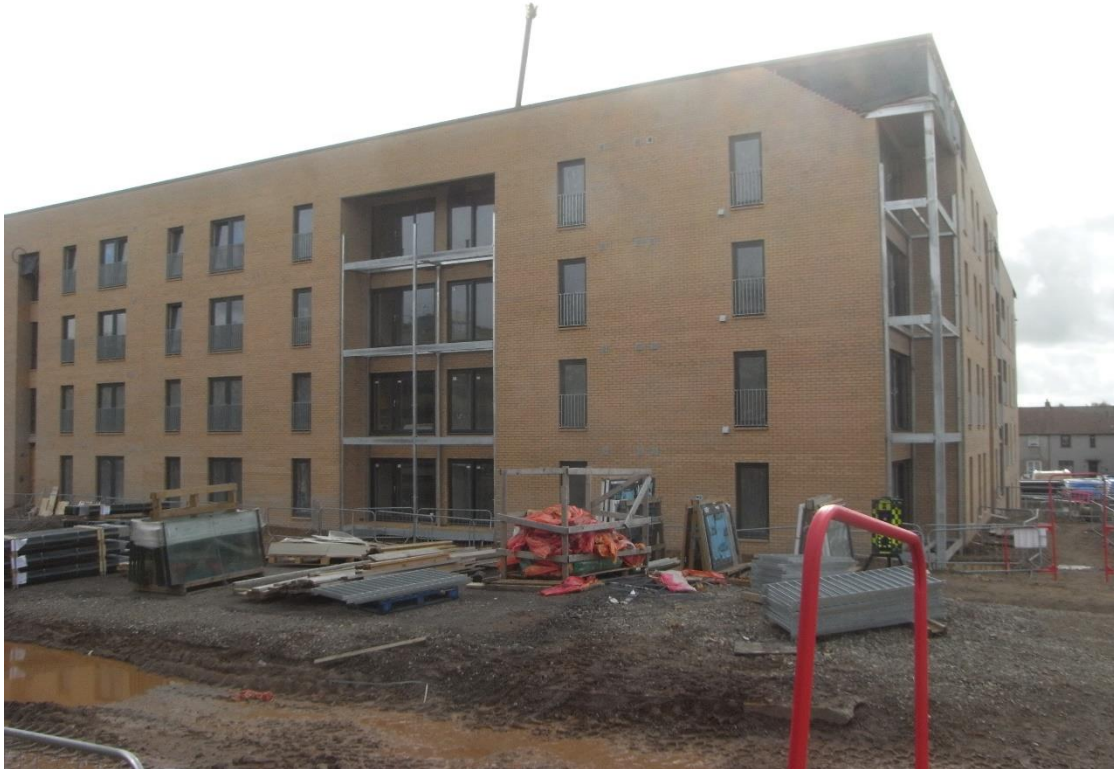
Block 5 – Balcony steelwork progressing (28.09. 2021)
