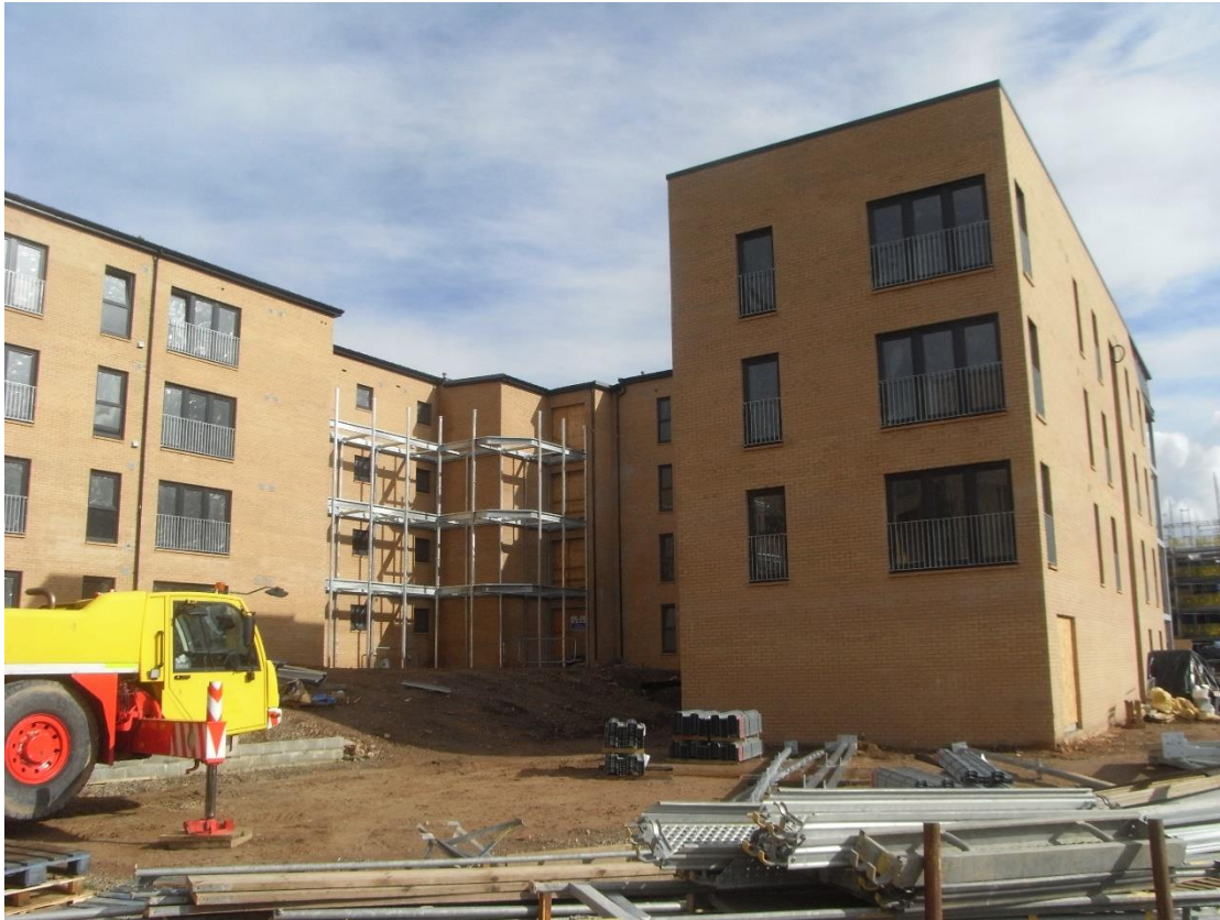
Block 5 – Completed Facing Brick; Installation of walkways (28.09.2021)
