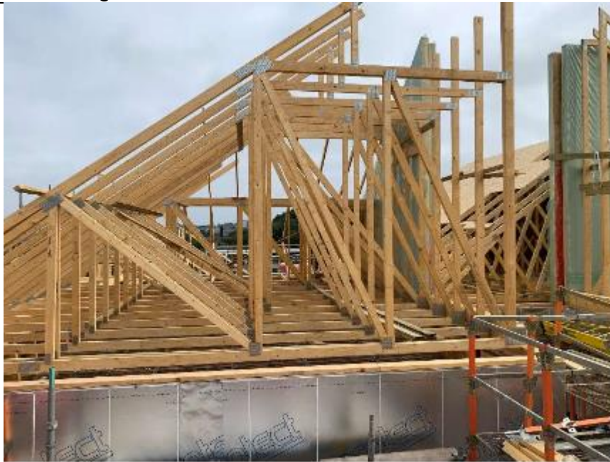
Roof trusses being installed – Block A
