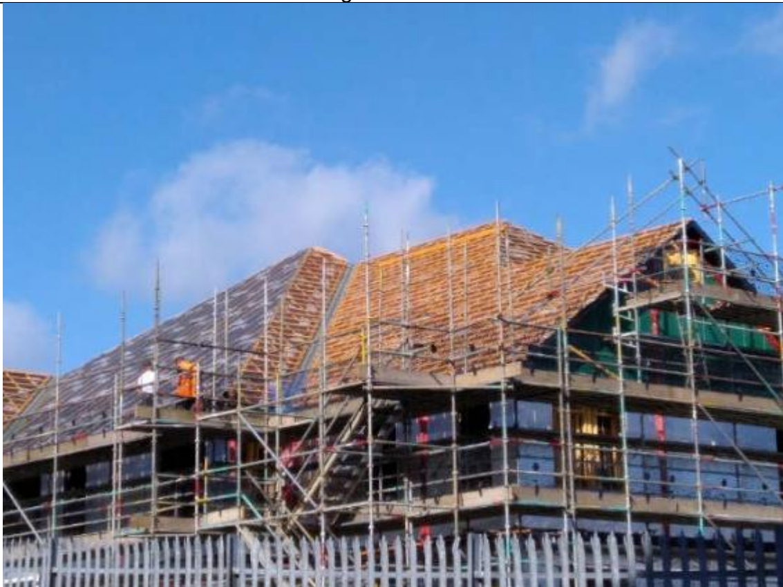
Block A Horizontal roof battens being installed
