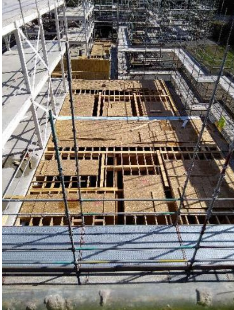
Block B 1 st Floor timber kit flooring being installed
