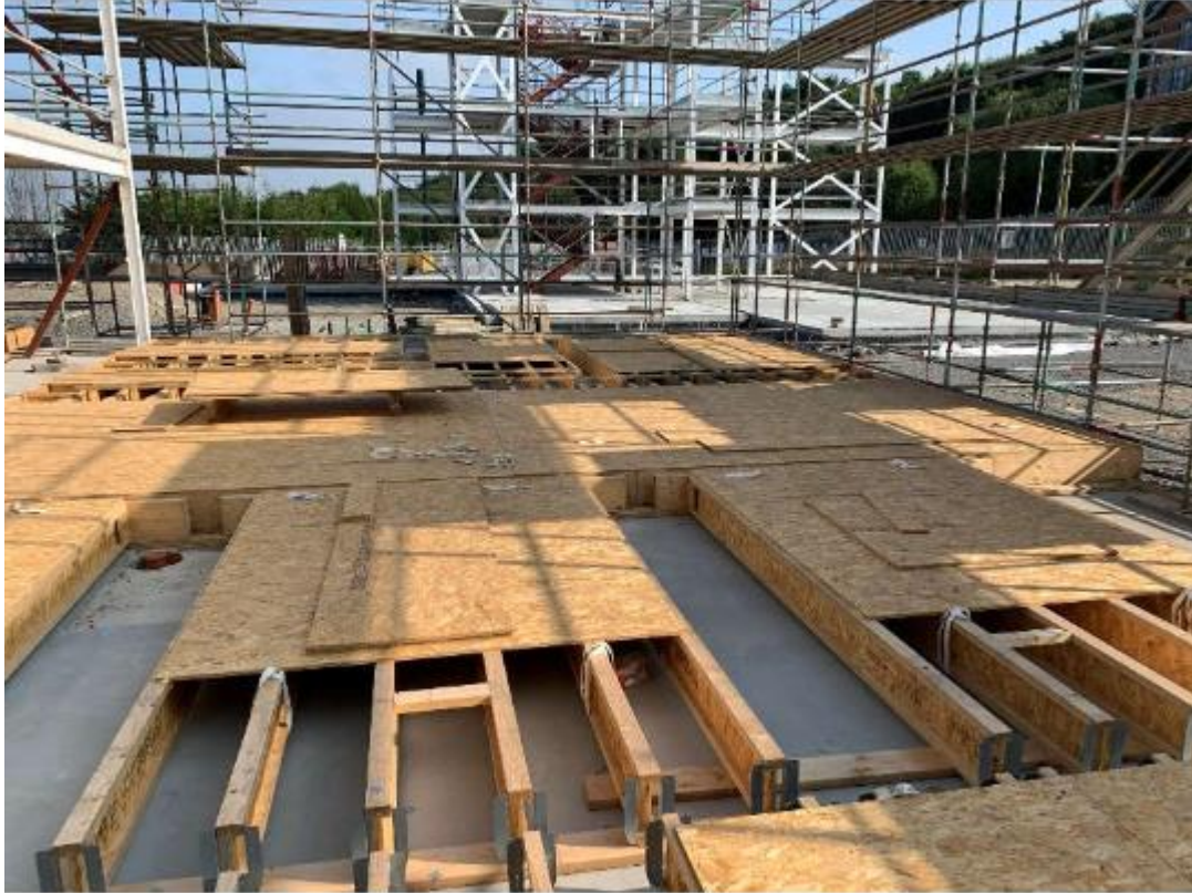
Cassettes for first floor formed on ground floor slab – Block B
